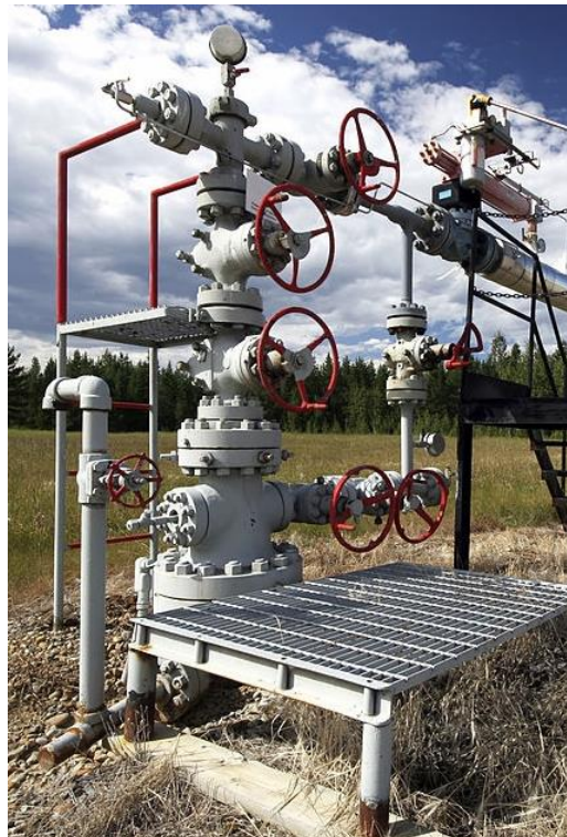
Figure 159 X-mass tree or Production tree
