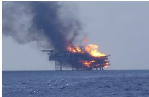
Figure 128 Blowout due to loss of control of formation pressure
