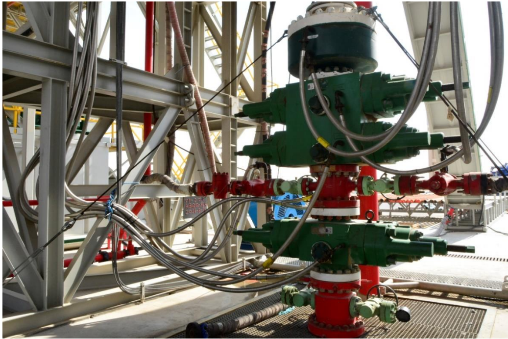
Figure 80 Blowout Preventer (BOP)
