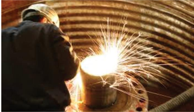
Figure 161 Cutting Casings
