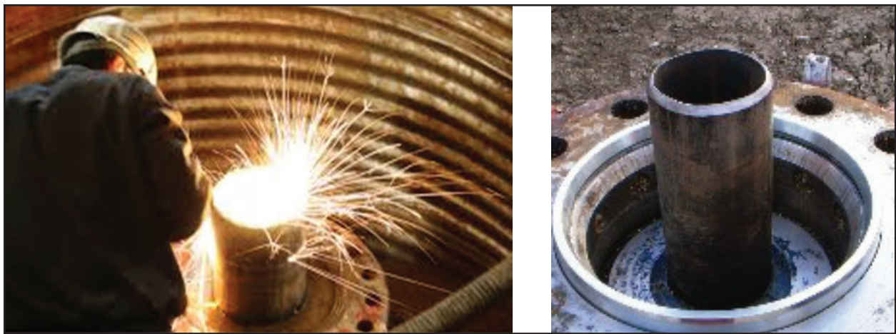
Figure 11 Casing Slip Assembly Set into Landing Base
